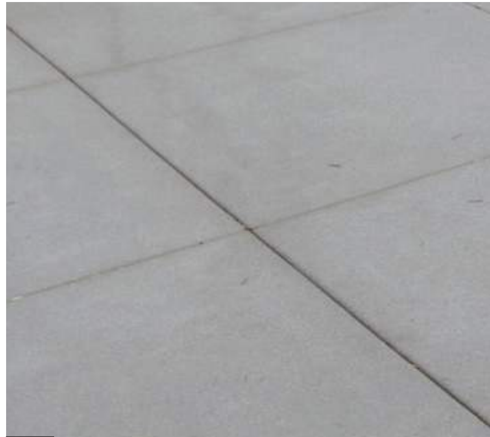
B SCORED CONCRETE PAVING
