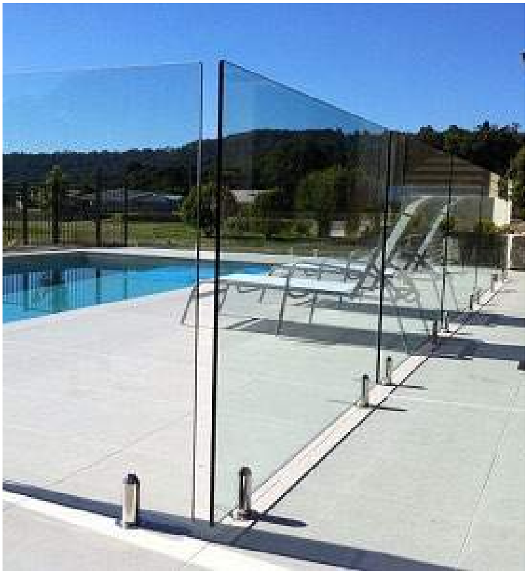
Pool Enclosure Glass Panels
