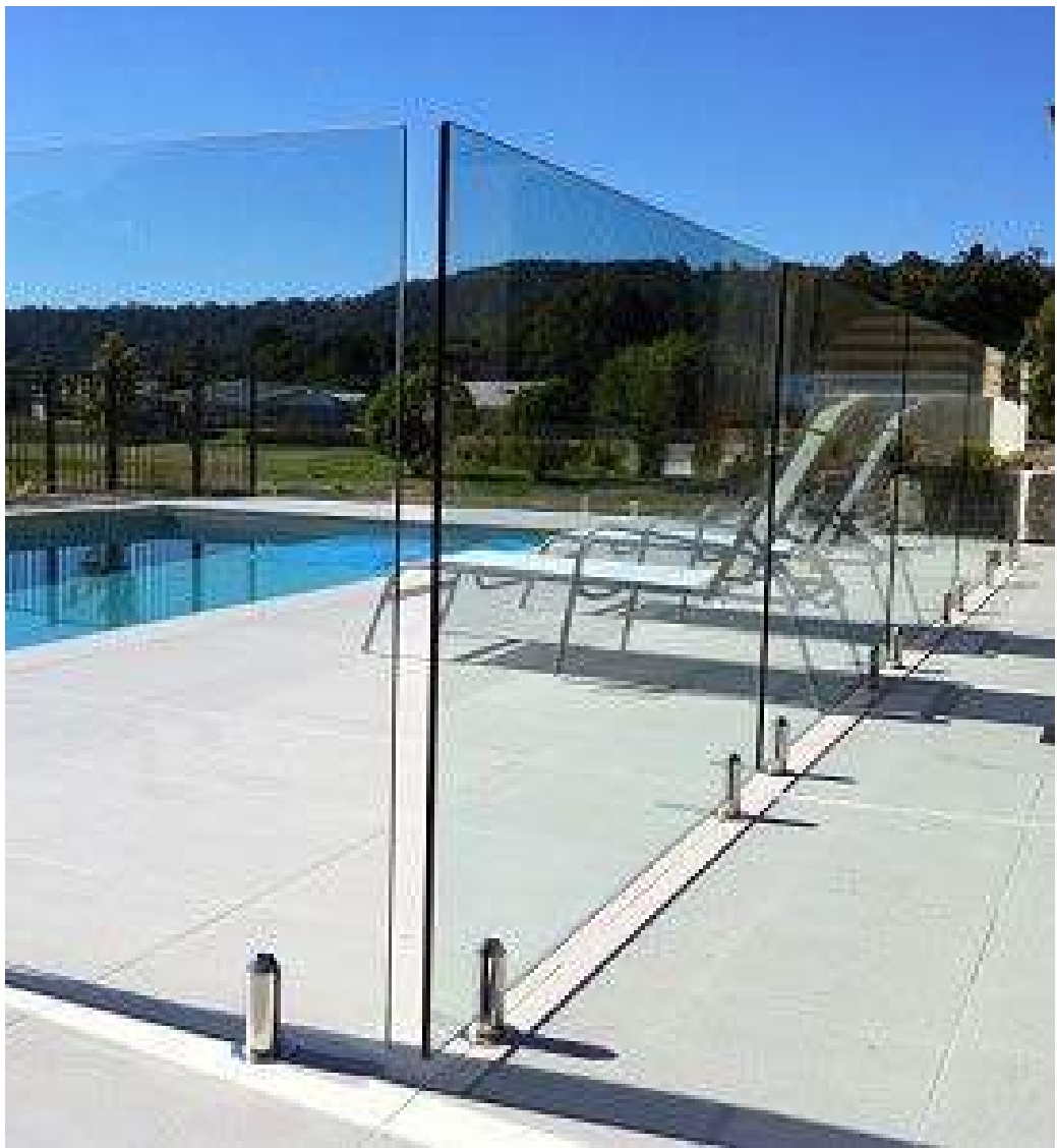
Pool Enclosure Glass Panels
